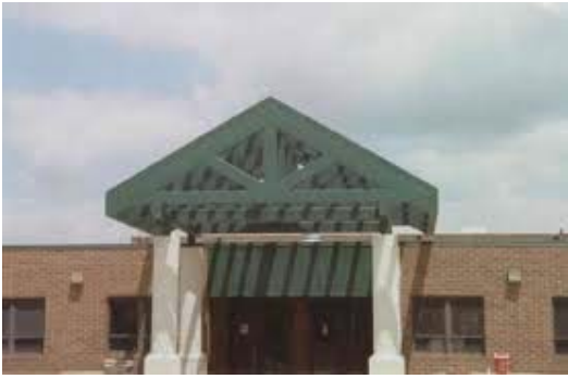
Pittsgrove Township Middle School
